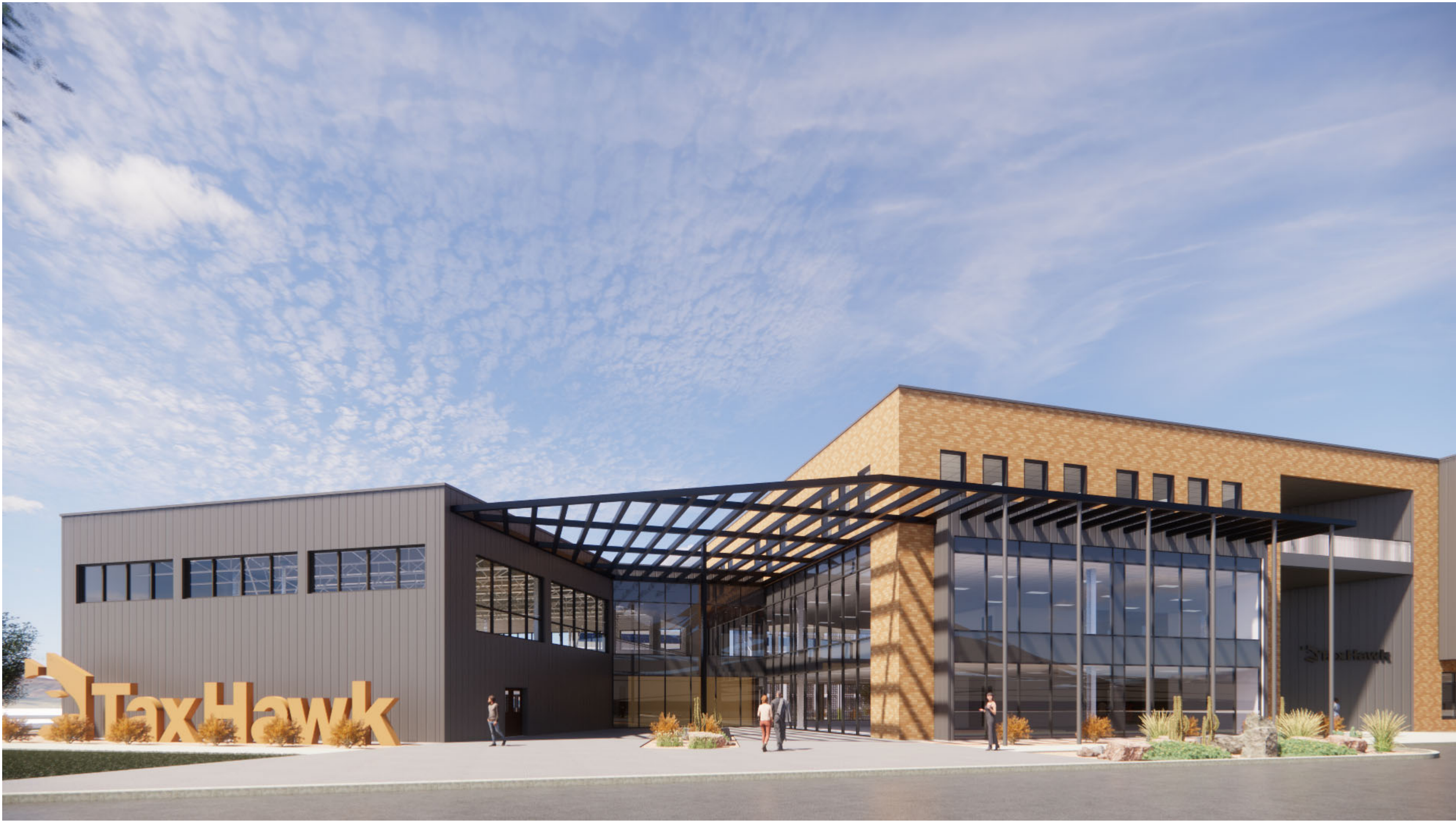
2. VIEW OF PLAZA FROM EAST DRIVEWAY
